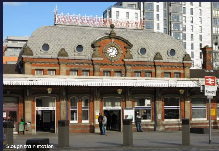
Slough train station
